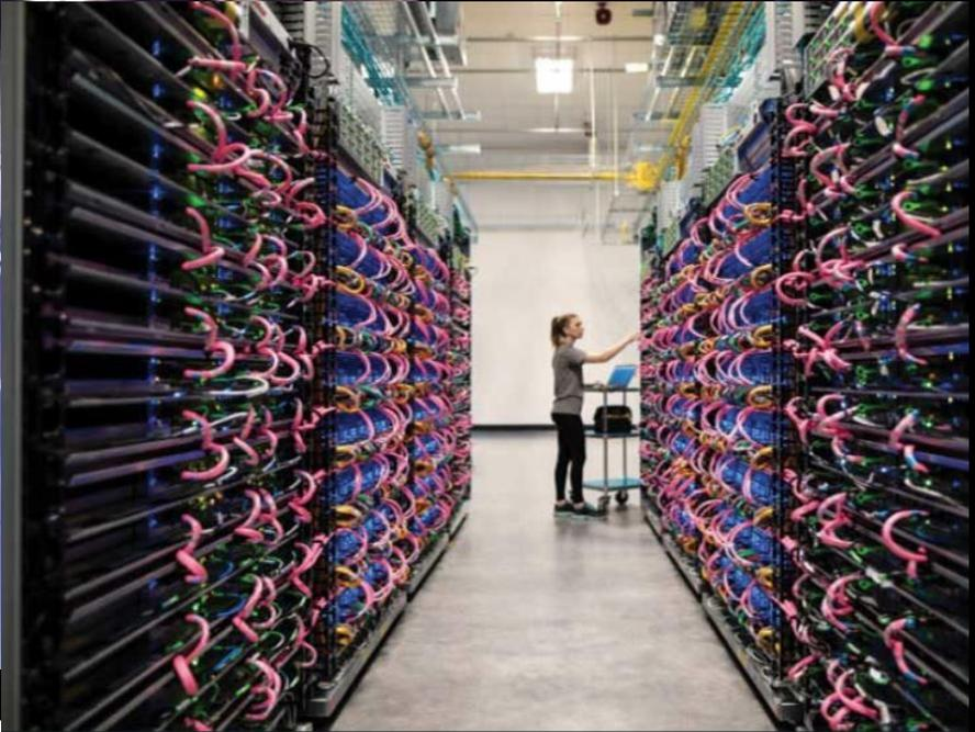
Google's liquid cooled TPU v2 servers deployed in racks. *Source: Google.*
